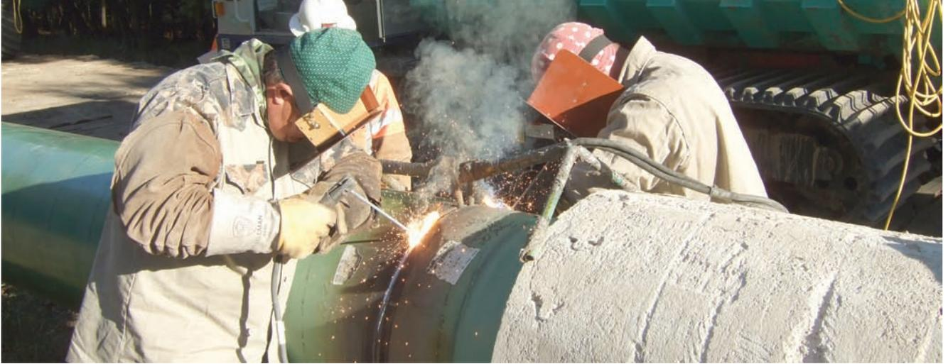
Today, high-strength steel pipe grades like X80 are widely used for long-distance transmission pipelines, but present a challenge for welding. In the past, field girth welds on X70 and lower strength grades were completed almost exclusively with cellulosic electrodes. However, with high-strength X80, cellulosic electrodes are typically only used for root and hot passes and not for fill passes due to the increased risk of HAC.
