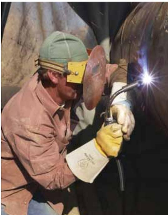
The use of Lincoln's STT GMAW solution not only offers productivity advantages, it also obviates the need to remove 'wagon tracks' associated with an SMAW root. This can significantly reduce the amount of rework required.
