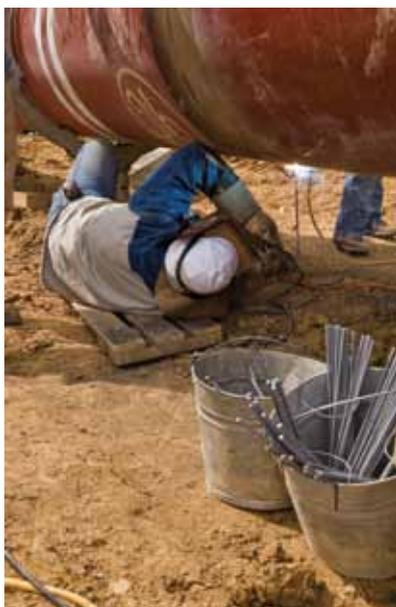
The use of Lincoln's true DC generators with its Pipeliner range of SMAW electrodes remains the most appropriate pipe welding solutions in many places of the world.
