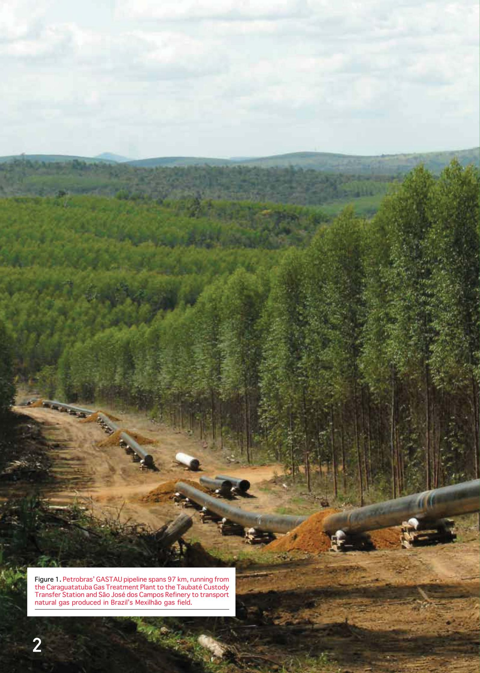
**Figure 1.** Petrobras' GASTAU pipeline spans 97 km, running from the Caraguatatuba Gas Treatment Plant to the Taubaté Custody Transfer Station and São José dos Campos Refinery to transport natural gas produced in Brazil's Mexilhão gas field.
