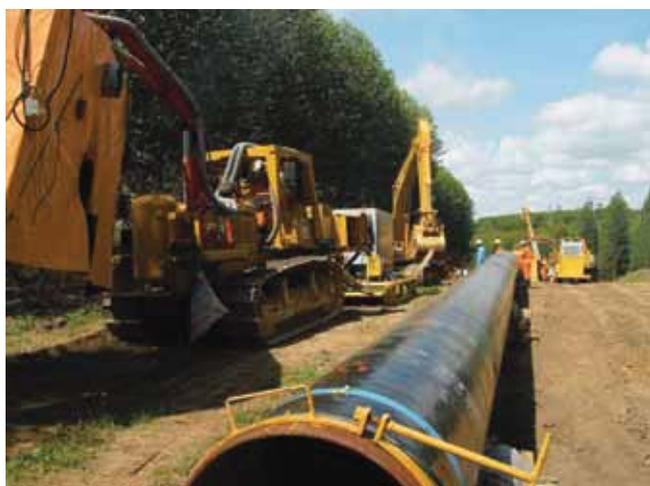
Figure 2. The GASTAU pipeline features 34 in. diameter (863 mm), 0.748 in. thick (19 mm) X80-grade pipe and is the first of this grade to be welded robotically in Brazil and the first to use Lincoln Electric's new Pipeliner® 80Ni1 welding wire.
